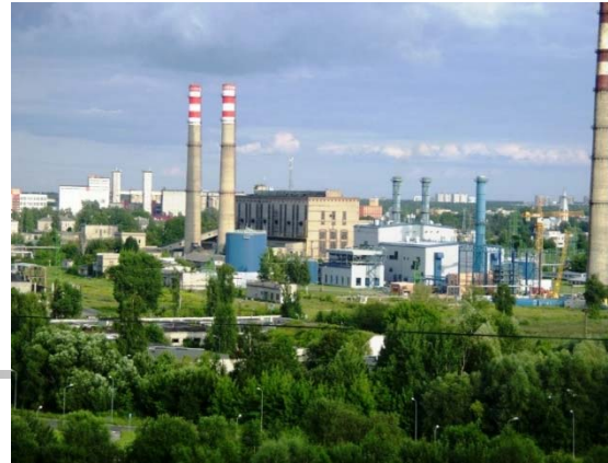
Riga CHP-1: (144 MWel, 493 MWth)
