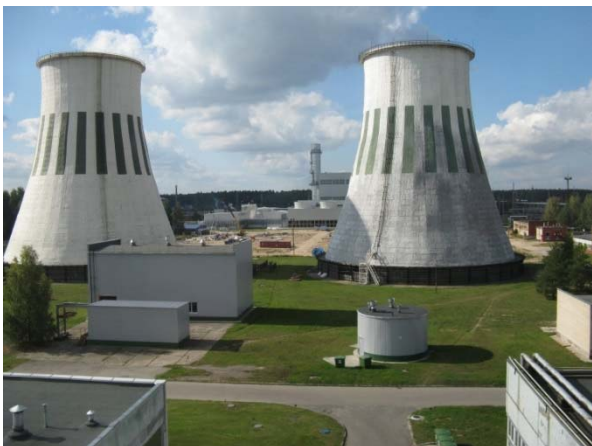
Riga CHP-2: (662 MWel, 1347 MWth)
