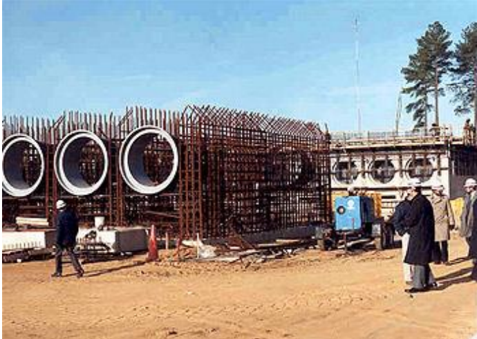
Horizontal casks being built
